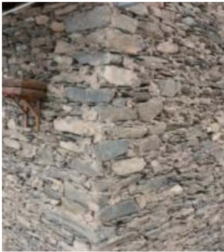
Figure 5: The corner block stones, Source: Research on Modern Pattern of Qiang Vernacular Dwellings in Region of Sichuan Province. Xi'an University of architecture and technology.
