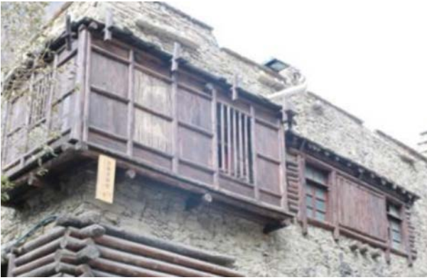
Figure 8: The external wooden room, Source: Research on Modern Pattern of Qiang Vernacular Dwellings in Region of Sichuan Province. Xi'an University of architecture and technology.
