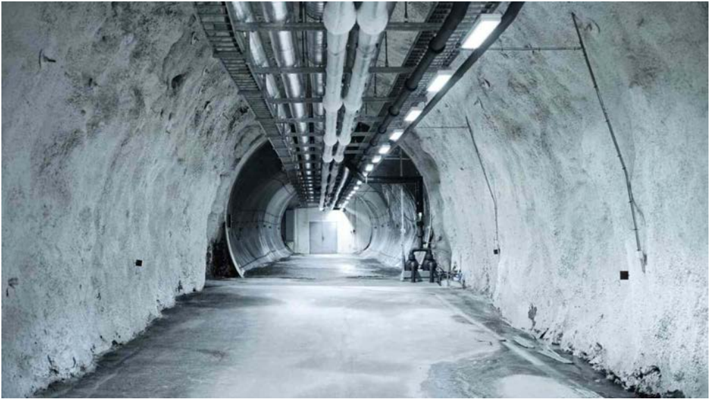
Figure 3: The entrance tunnel. Svalbard Global Seed Vault, Norway, 2008. Ph. Matthias Heyde
