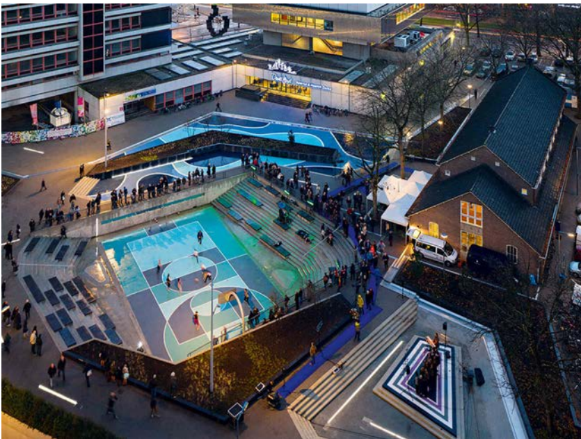
Figure 2: Bentheplein in Rotterdam. The image shows sequence of the three main basins, which are normally used for recreational purposes but can be transformed into water storage during extreme weather conditions. Source: https://www.theneweconomy.com/technology/rotterdams-water-management-gives-rise-to-exceptional-city (accessed June 2021)
