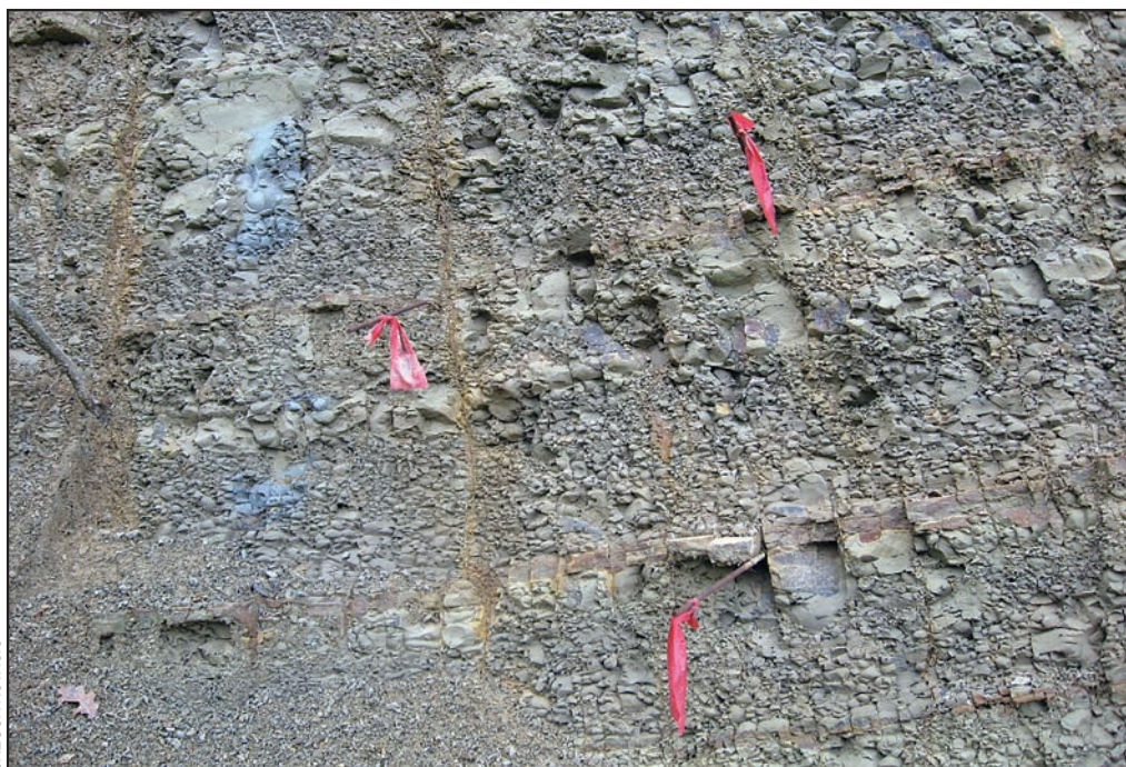
Figure 5: Erosion pins for direct measurements of flysch cliff retreat, April 28 th , 2008.
