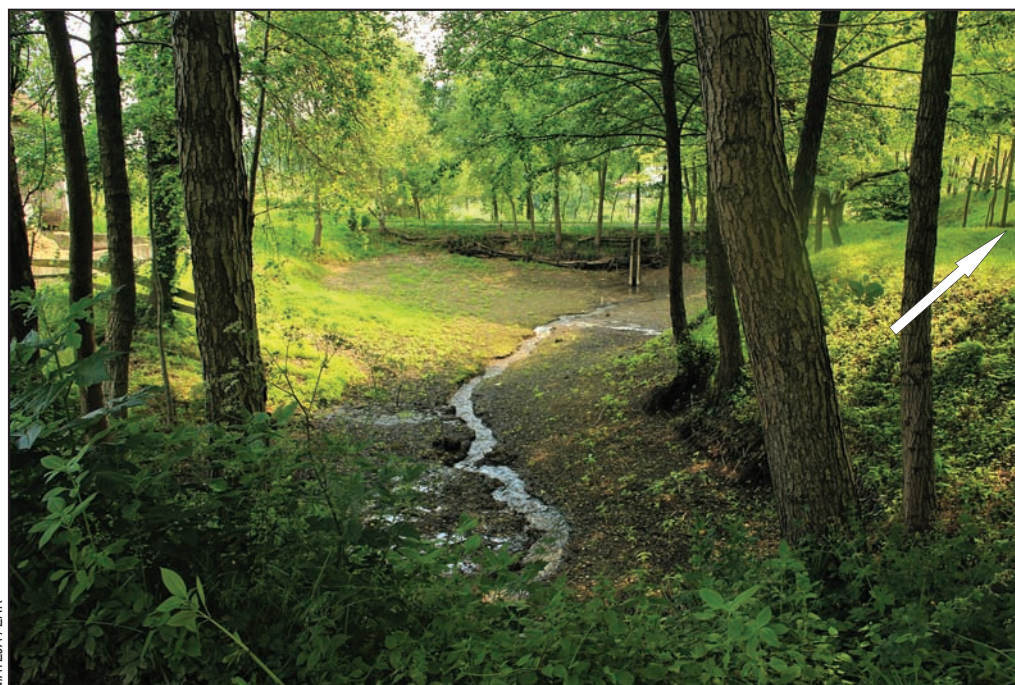
Figure 5: Vegetation is removed from the banks of the retention ponds every few years. White arrow is indicating the location of the diversion channel which diverts the excess water and bedload around the pond.
