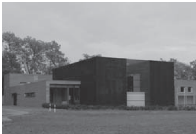
Slika 4: Prva cerkev v pasivnem standardu, Wels, Avstrija. Figure 4: First church built according to passive standards, Wels, Austria.
