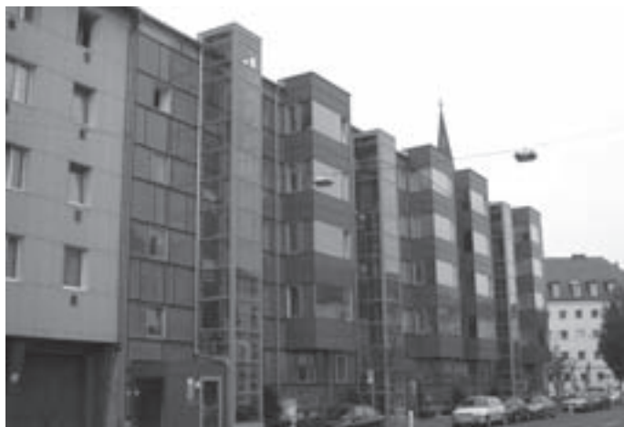
Slika 11: Sanacija večstanovanjskega objekta v pasivnega, Linz, Avstrija. Figure 11: Remediation of a multi-occupied building and conversion into a passive one, Linz, Austria.
