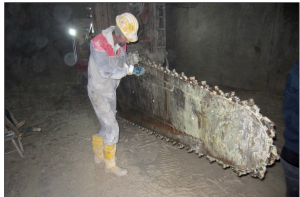
Figure 4. Diamond wire and chain cutting machine.
