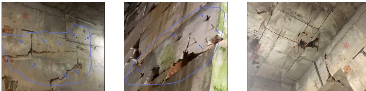
Figure 7. Different types of pillar discontinuities.
