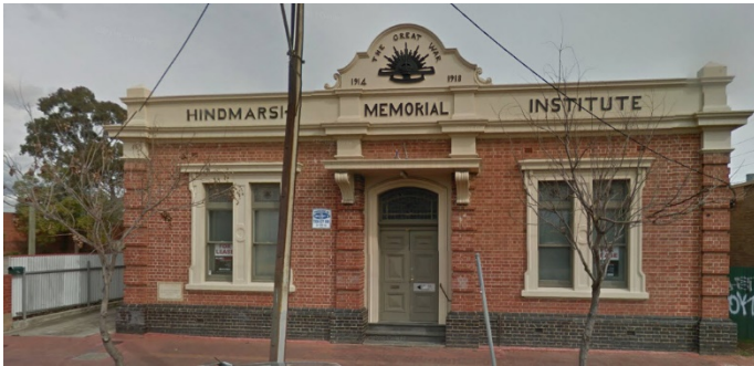
Hindmarsh Memorial Institute, 262 Port Road, Hindmarsh, 5007.
