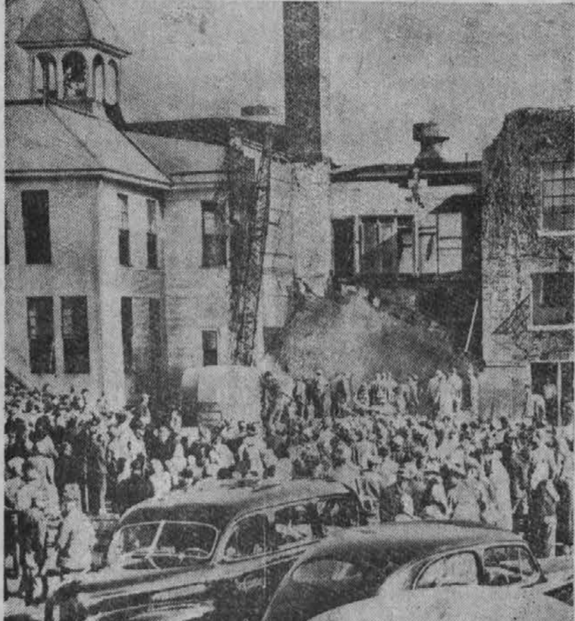
BLAST WRECKS SCHOOL . . . Crowds of anxious parents and volunteer rescue workers gathered quickly at the Baroda consolidated school at Baroda, Mich., following a boiler explosion in the basement of the school which killed one child and injured at least 16 others. When reports were first received at Chicago rescue planes with medical supplies were rushed to the scene.
