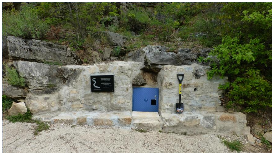
Figure 1. The completed protected entrance to the »Trebinje Proteus Observatory« at the Vrelo »Vruljak 2« cave (photo: B. Lewarne).
