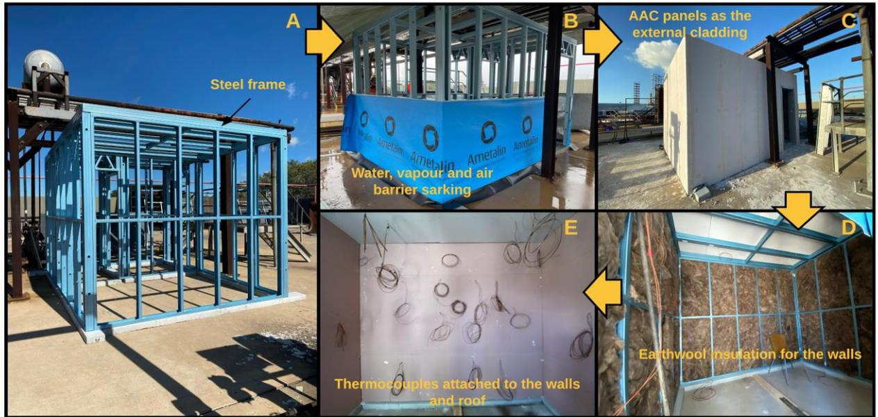
Fig. 1 Construction sequence of the safe room
