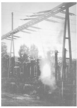
Fig. 2. Standing arc in a substation switchgear
