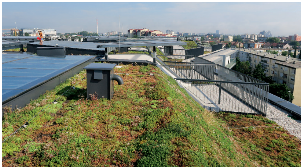
Figure 1: Green roof in Ljubljana.
