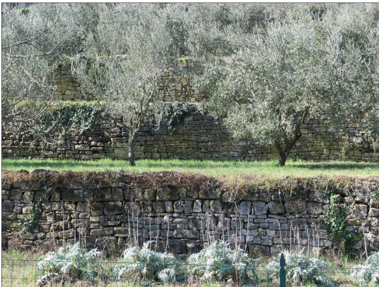
Figure 8: Traditional terraces in northern Istria (Strunjan) with dry stone embankments (Photo: Darko Likar)
