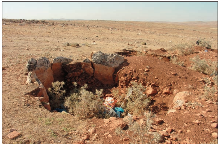
Fig. 4. Building was found in a stable condition, with only its interior part approaching bed rock being destroyed.
