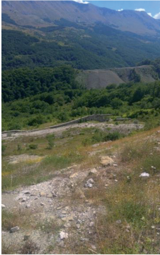
Figure 4: The landslide "ČemernskoOsoje".
