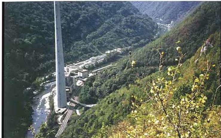
Slika 2: Termoelektrarna Trbovlje Figure 2: Trbovlje steam power station
