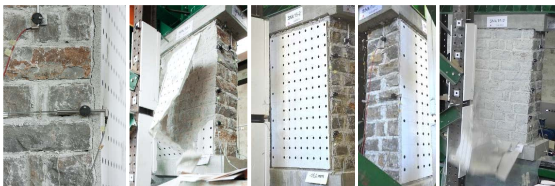
Figure 3.74: Detachment and collapse of the plaster at test 12 - SPk-15-1 (left two) and 14 - SNk-15-2 (right three) Slika 3.74: Odstopanje in porušitev ometa pri testu 12 - SPk-15-1 (levi dve sliki) in testu 14 - SNk-15-2 (desne tri)
