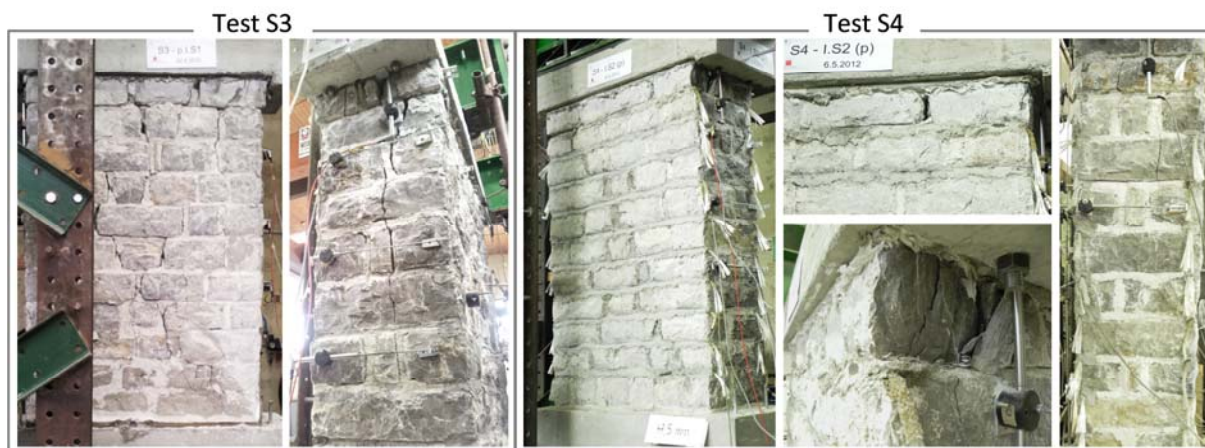
Figure 5.14: Rocking and minor shear damage on the wall after test S3 – I.S1(p) and rocking and toe crushing at test S4 - I.S2(p)
