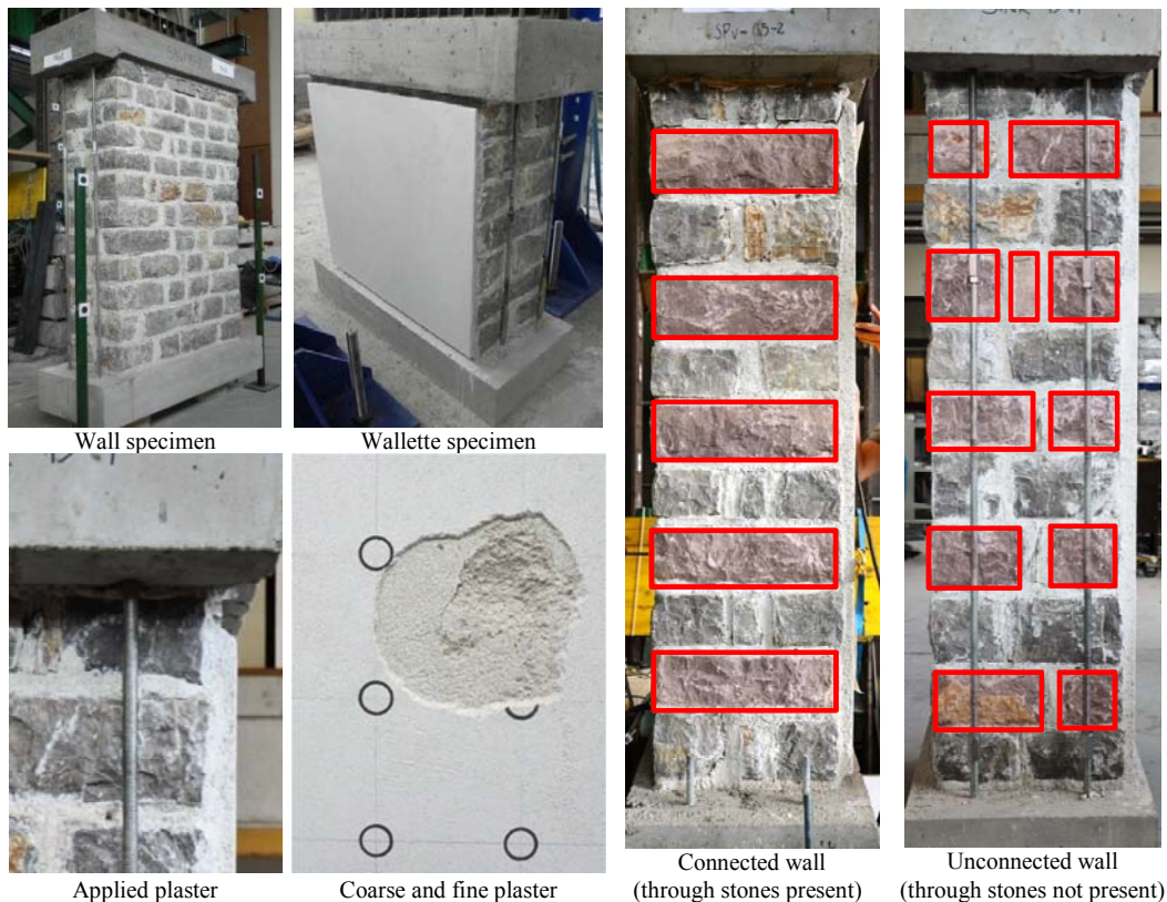
Figure 3.5: Different wall specimens; side view and the applied lime plaster - coarse and fine layer
