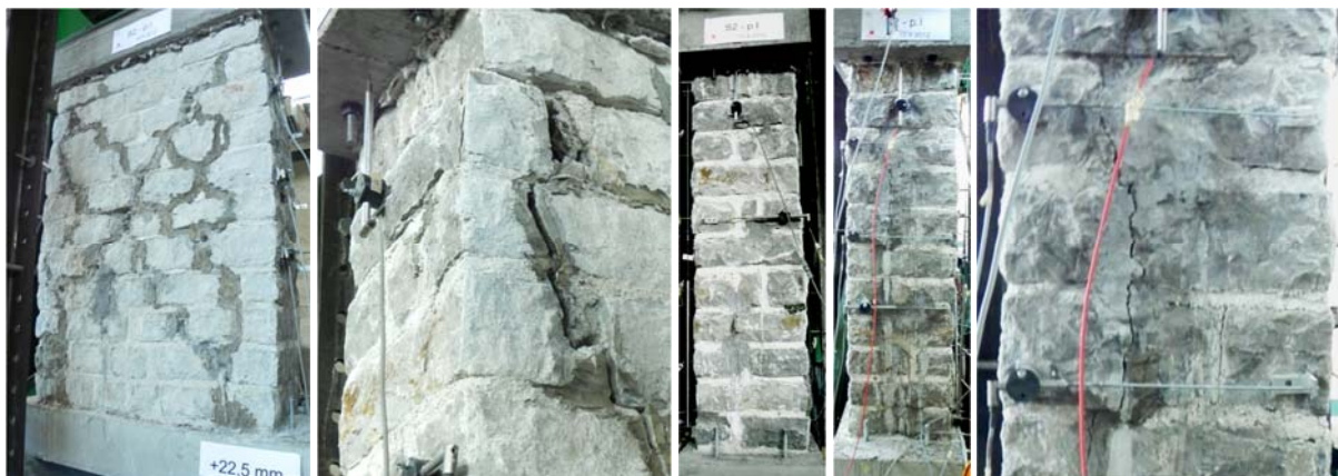
Figure 5.13: Damage after test S2 – I(p) on the front and transversal sides of the wall Slika 5.13: Razpokanost zidu na prednji in stranskih straneh zidu po testu S2 – I (p)
