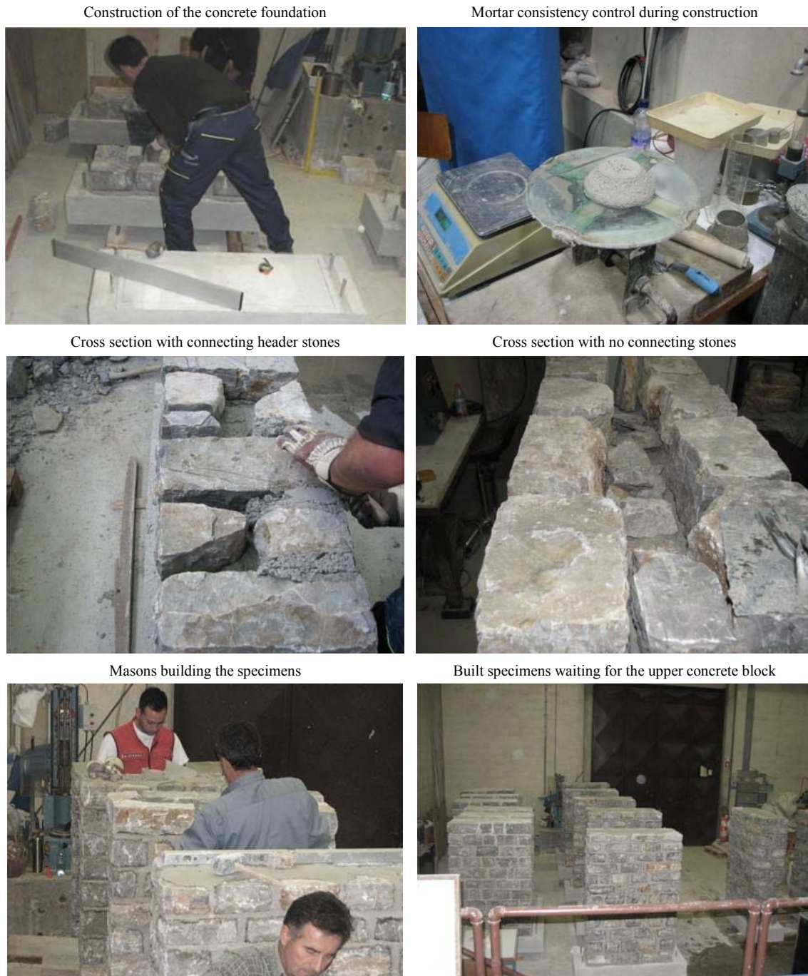
Figure 3.2: Construction of the specimens
