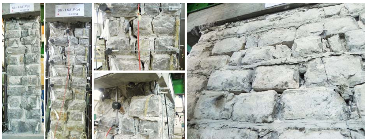
Figure 5.17: Leaf separation, toe-crushing damage and cord detachment with partially emptied mortar joints after test S6 - I.S2-.P (n)
