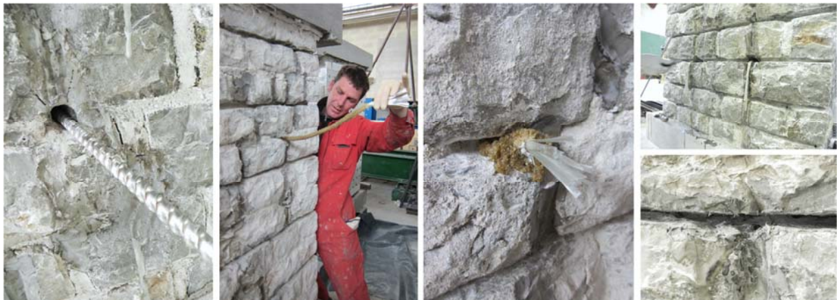
Figure 4.18: Drilling of the hole, the insertion of the impregnated cord coated in sand and sand "plug", transversal connection with impregnated cord (upper right) and with spread and fixed fibres (test 8 only, bottom right) Slika 4.18: Vrtanje luknje, povezovanje slojev zidu z impregnirano in s peskom posuto vrstico, pečeni "čep", prečna povezava z impregnirano vrstico (zgoraj desno) in razprostrta in prilepljena vlakna (samo test 8, spodaj desno)
