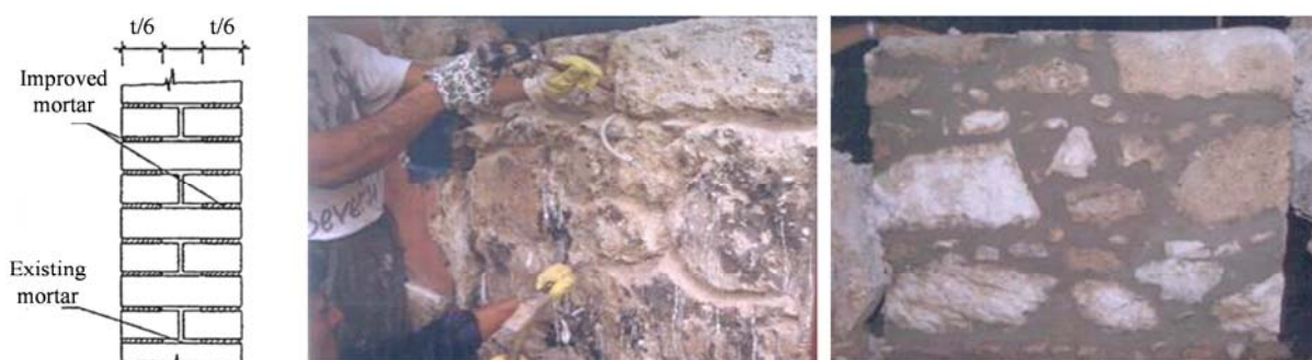
Figure 2.25: Deep repointing of brick (left, adapted from [168]) and of stone masonry (middle and right) [170] Slika 2.25: Prefugiranje opečne (levo, prilagojena [168]) in kamnite zidovine (na sredini in desno) [170]
