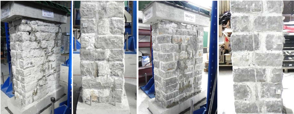
Figure 5.1: Grouted wall with existing damage pattern prior testing (test T1 - I(n)) Slika 5.1: Injektirani zid z obstoječimi razpokami pred testiranjem (test T1 - I(n))
