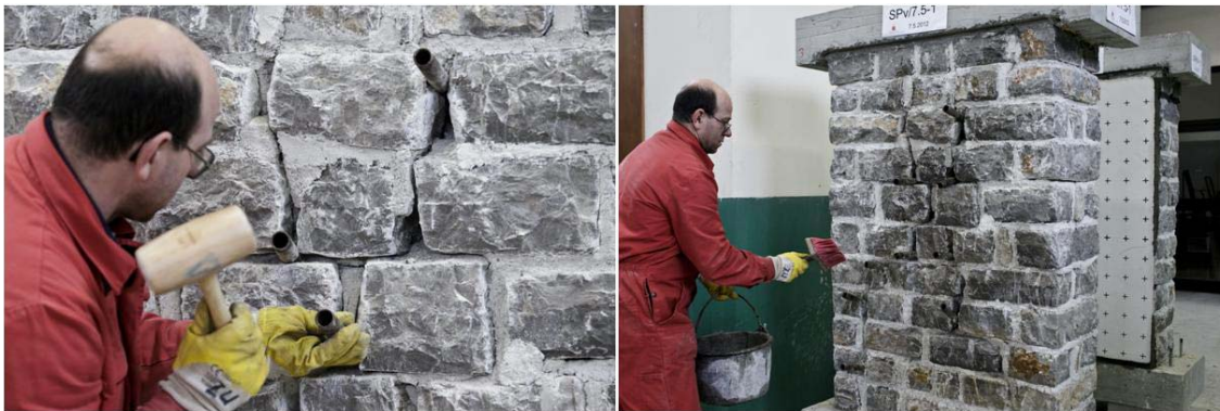
Figure 4.12: Inserting tubes (left) and pre-wetting the wall (right) (photos Željko Stevanić for UL FGG) Slika 4.12: Umeščanje cevk v zidove (levo) in vlaženje zidu (desno) (foto Željko Stevanić for UL FGG)
