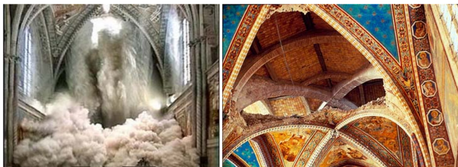
Figure 1.4: Collapse of the St Francis of Assisi Basilica ceiling during 1997 Umbria-Marche earthquakes (left, http://projecthistoryitalia.altervista.org/26-settembre-1997-terremoto-nelle-marche-e-in-umbria/ ), destroyed Cimabue fresco vault ceiling in the Assisi Basilica (right, http://it.wikipedia.org/wiki/File:Volta_Cimabue.jpg )
