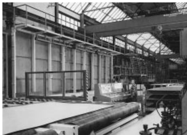
Figure 3: Vertical spray pickling plant at Krupp VDM with solid metal segments in alloy 31 in highly stressed areas
