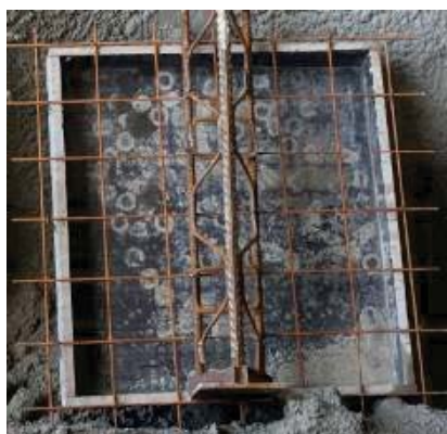
Kalup z vgrajenim lokom in armaturo
