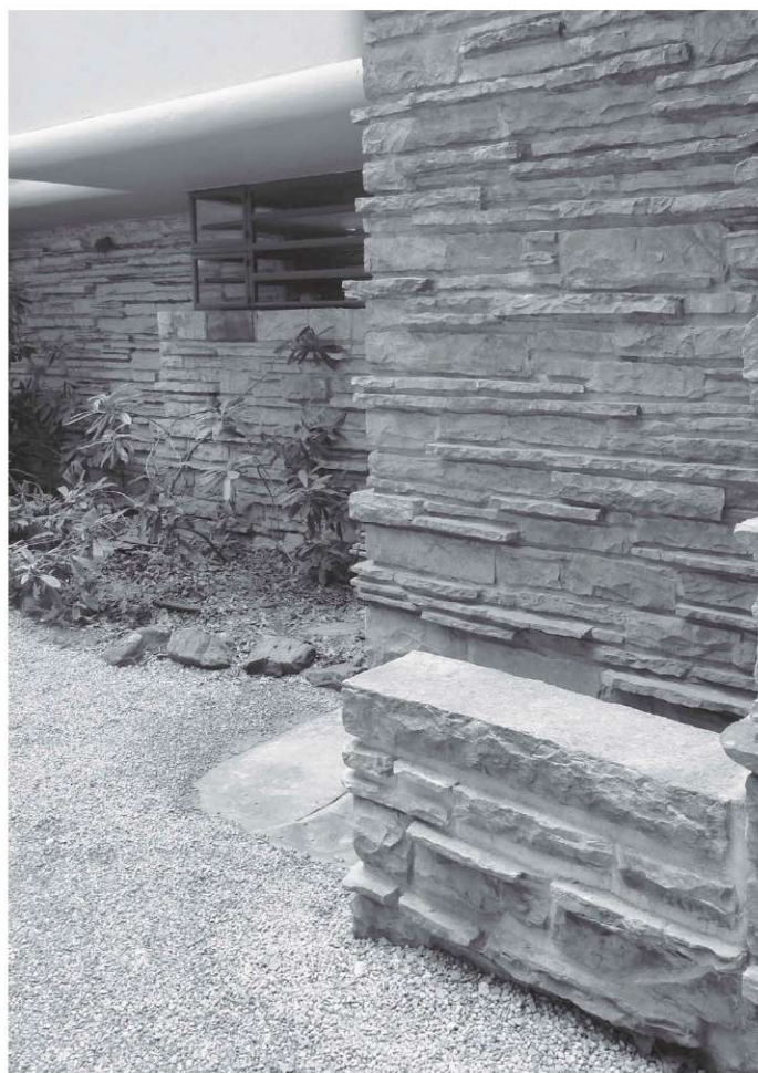
Slika 5: Fallingwater – vodoravno naložen kamen ponazarja plasti naravnega peščenjaka. Figure 5: Fallingwater – the horizontally laid stone illustrates the strata of natural sandstone.
