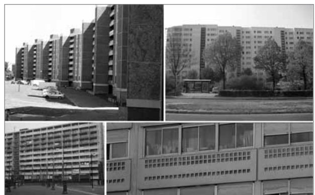
Figure 2: High-rise estates under reconstruction (photo: Pascal De Decker and Caroline Newton).
