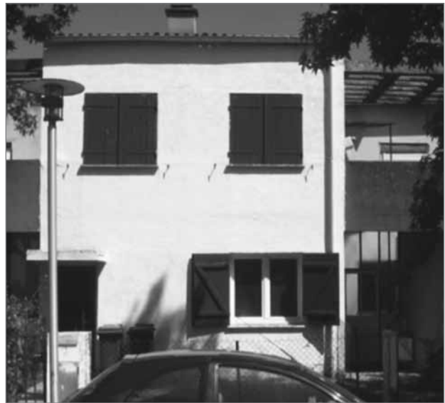
Figure 5: Pessac today – note the alterations made by the inhabitants (source: Internet 1).
