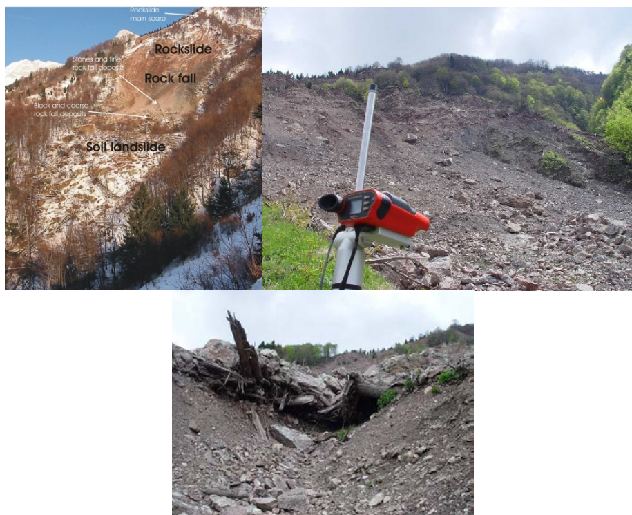
Figure 10: The complex Strug Landslide: photo taken on 31 December 2001 (upper left); an upslope view of the rock fall source area towards the crown (upper right); a new gully was measured in May 2004 (bottom).
