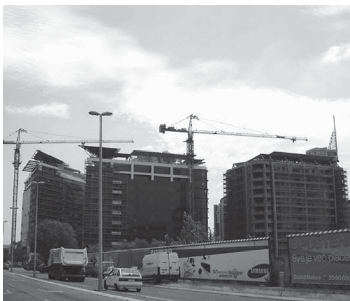
Figure 7: Novi Beograd building site, 2008, photo made by author. Slika 7: Gradbišće v Novem Beogradu, 2008.
