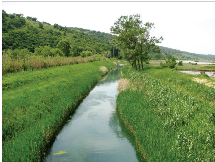
Figure 1: Embankments along the lower section of the Dragonja River
