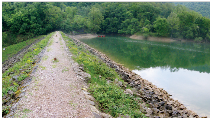
Figure 2: Vanganel detention reservoir on the Bavški potok torrent in the drainage basin of Badaševica
