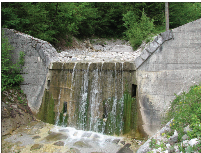
Figure 3: Check dam constructed on the Bistričica torrent
