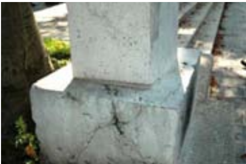
Slika 4: Spojnica med trupom in bazo Gallusove herme, Vegova ulica. The bond between the body and base of Gallus's herma, Vegova Street.
