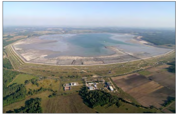
Figure 1. General view of the OUOW Żelazny Most [KGHM Polska Miedz S.A.].
