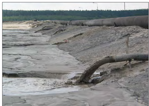
Figure 2. Spigotting of post-flotation tailings at the Żelazny Most depository.
