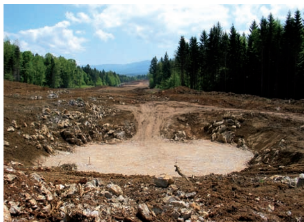
Fig. 4: Filling of dolina with gravel.
