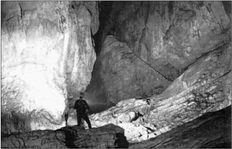
Fig. 9: Steps cut in the rock by the Section Küstenland. View from Rudolf Dom looking downstream. The shallow steps on right in the middle distances are the earliest, dating probably from 1884 or 1885. The steep steps in the background were perhaps made in preparation for the tourist route extending to Müller Dom in 1890. (photo A. Mihevc).
