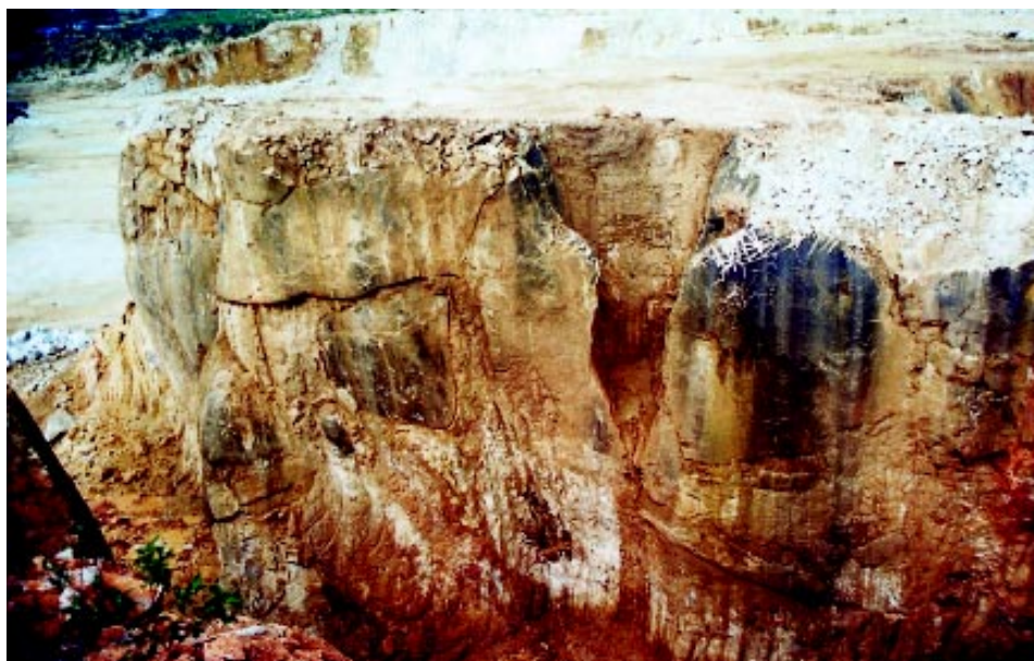
Fig. 4: The shape of walls of karst depression after fill was removed, note overhanging walls, Velkolom Čertovy schody-Quarry East (Photo by P. Bosák, September 1994).
